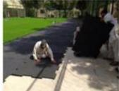
Type: EPP(Expanded Polypropylene) Foam Shock pad
